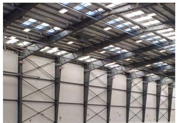
The minimum W/D should be specified for alternative fire protection assemblies, in addition to the structural criteria.
