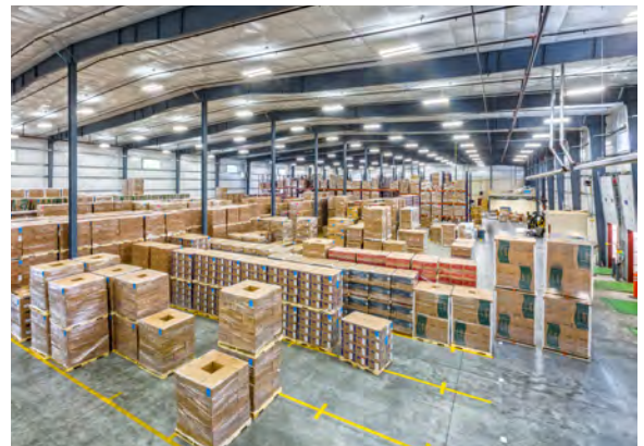
Fire protection using SFRM and intumescent coatings can be considered where a finished interior appearance with gypsum board is not necessary, such as industrial and warehouse buildings.
