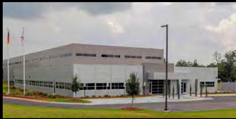
MANUFACTURING/INDUSTRIAL BERGHOFF PRECISION MACHINING, LP LOCATION / Auburn, Alabama BUILDER / Bailey-Harris Construction ERECTOR / Caraway Steel ARCHITECT / Terry Doyle / Black Design Architecture
