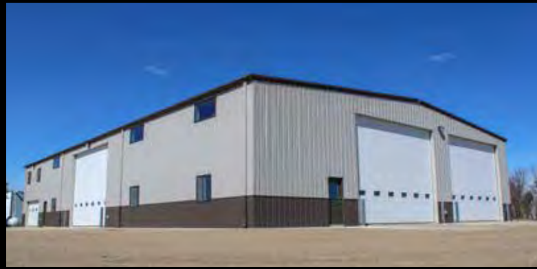
AGRICULTURAL BOEKELHEIDE & SONS, INC. LOCATION / Northville, South Dakota BUILDER / Tailored Structures, LLC
