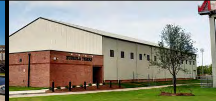
RECREATION EUFULA HIGH SCHOOL ATHLETIC SPORTS COMPLEX LOCATION / Eufaula, Alabama BUILDER / Anderson Construction Co. of Fort Gaines ERECTOR / Ustry Construction ARCHITECT / Blondheim & Mixon, Inc.
