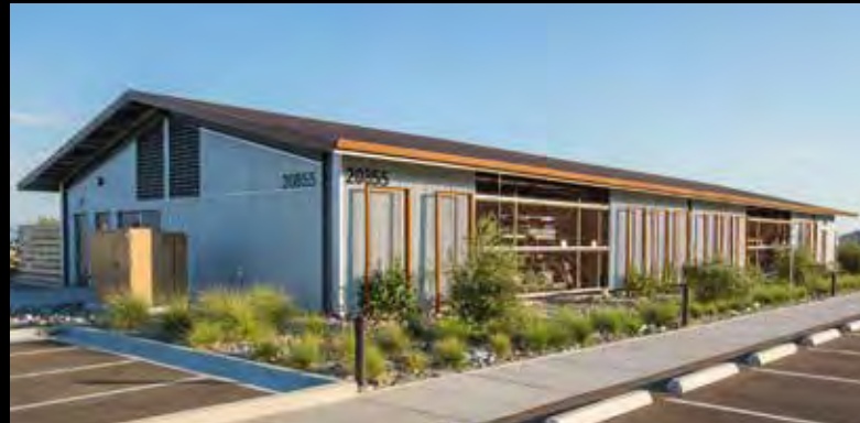
RECREATION VERRADO GOLF CLUB - GOLF CART BARN LOCATION / Verrado, Arizona BUILDER / Colton Constructors ARCHITECT / SHJ Studio
