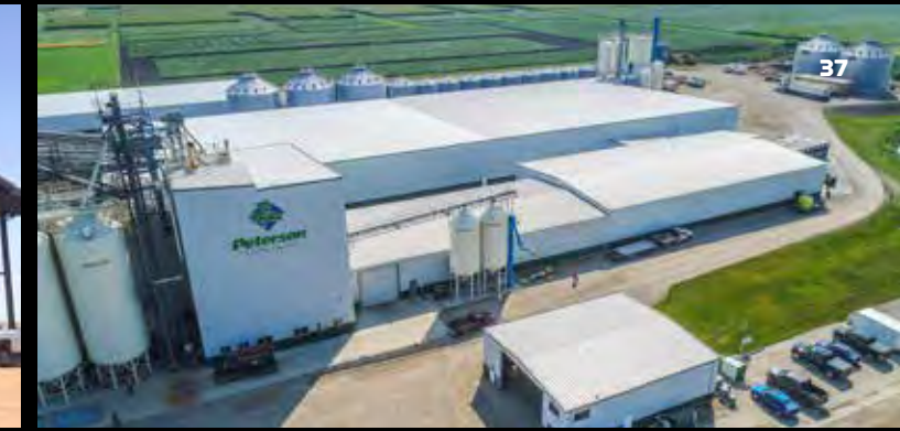
AGRICULTURAL PETERSON FARMS SEED LOCATION / Harwood, North Dakota BUILDER / Pfau Steel Buildings
