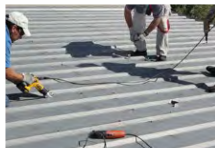
1. Cut out roof.
