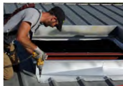
3. Install roof curb.
